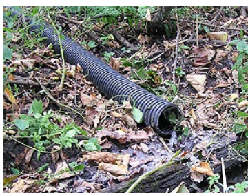
Straight pipe discharge of wastewater.
